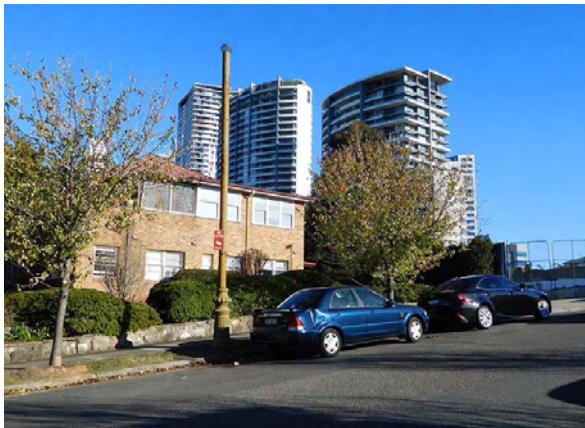
11 View south-west from Wilson Street - Chatswood CBD towers visually prominent and form urban backdrop
