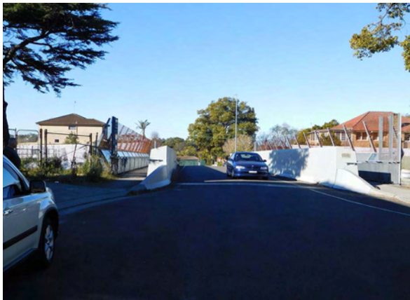
14 View east across the Wilson Street rail bridge towards the site
