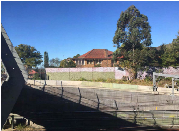
15 View west from Wilson Street across railway line - safety / retaining wall forms prominent visual element along boundary
